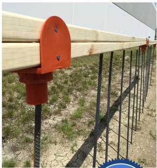
Each Impalement Safety Cap is stamped with the California OSHA approval number as required by CAL-OSHA.
